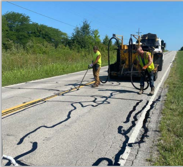
Pavement Management Contractors – Crack Sealing
